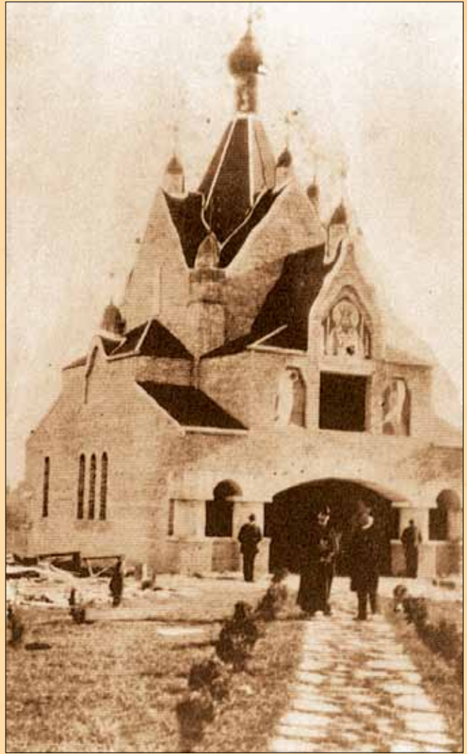
St. Sava Church in Libertyville during construction
